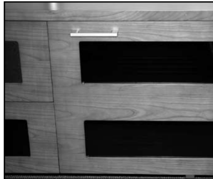
CORRECT! Door is sitting squarely and evenly spaced on tops and sides.
